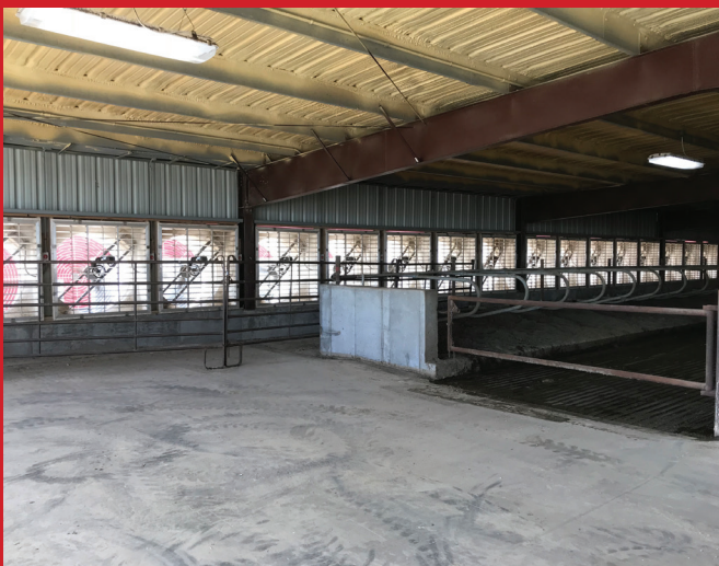
Freestall Barn Ventilation
